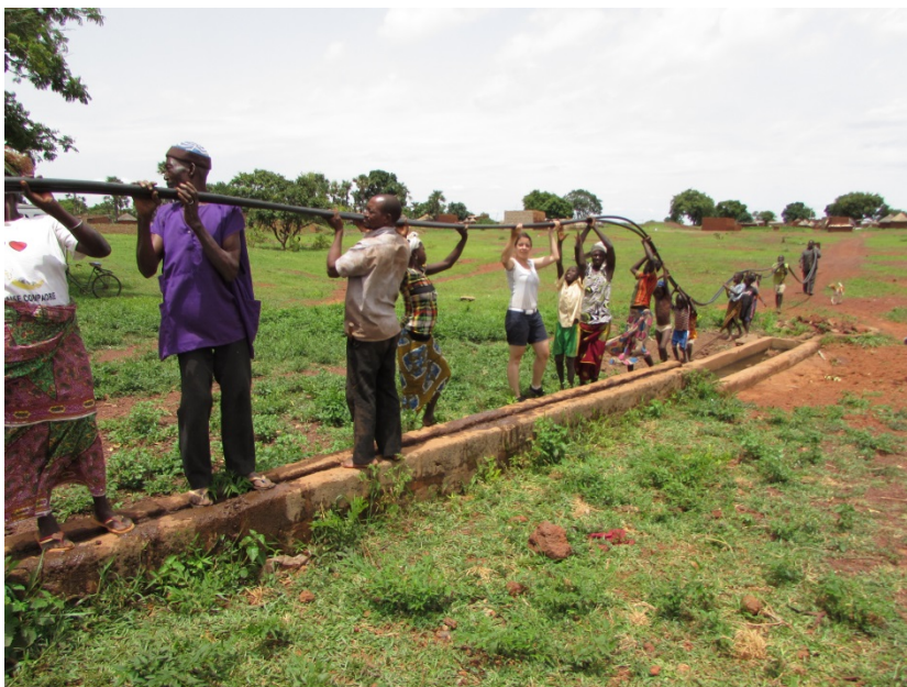
'Helping Hands' assisting with the well repairs at Noumoudara
