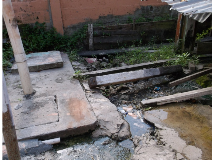
Drainage Before (top)
