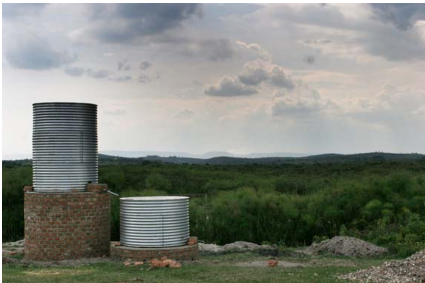
Water treatment/storage structure constructed beside local water source.
