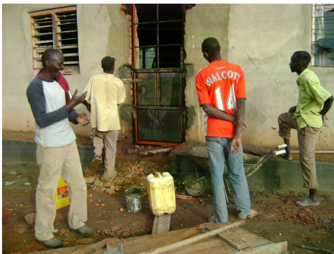
Fixing the door of the Library during the renovation process.
