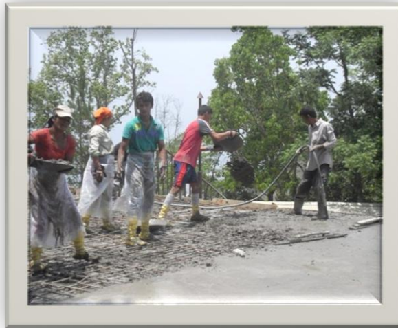
Local labor workers building the concrete roof for completing six new classrooms
