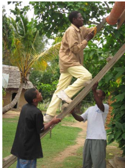
Installing a rain water catchments system
