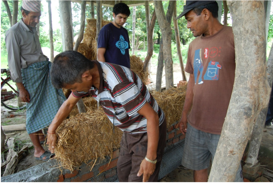
(Left) Raising an inside wall of the building in Shivagadi
