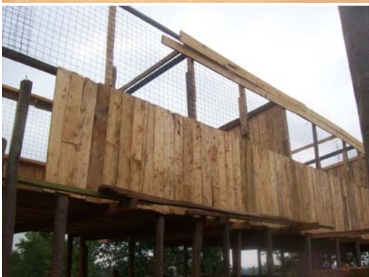
The double-storey poultry farm, soon to accommodate over a hundred chickens.
